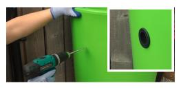
**b.** Using a 32mm hole-saw or spade bit provided, cut a hole just below the base of the planter bowl and insert the rubber seal.
