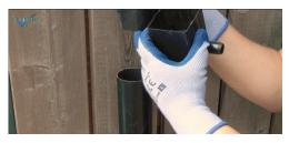
**Note:** The pipe between the downpipe and the water butt <u>must</u> be horizontal.
