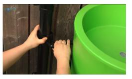
e. If, when fixing a tap to the raised outlet, the tap does not face downwards, use another layer of PTFE and try again. Do not use too much tape as this may damage the threaded outlet. Hand tighten only; do not use a spanner or wrench.
